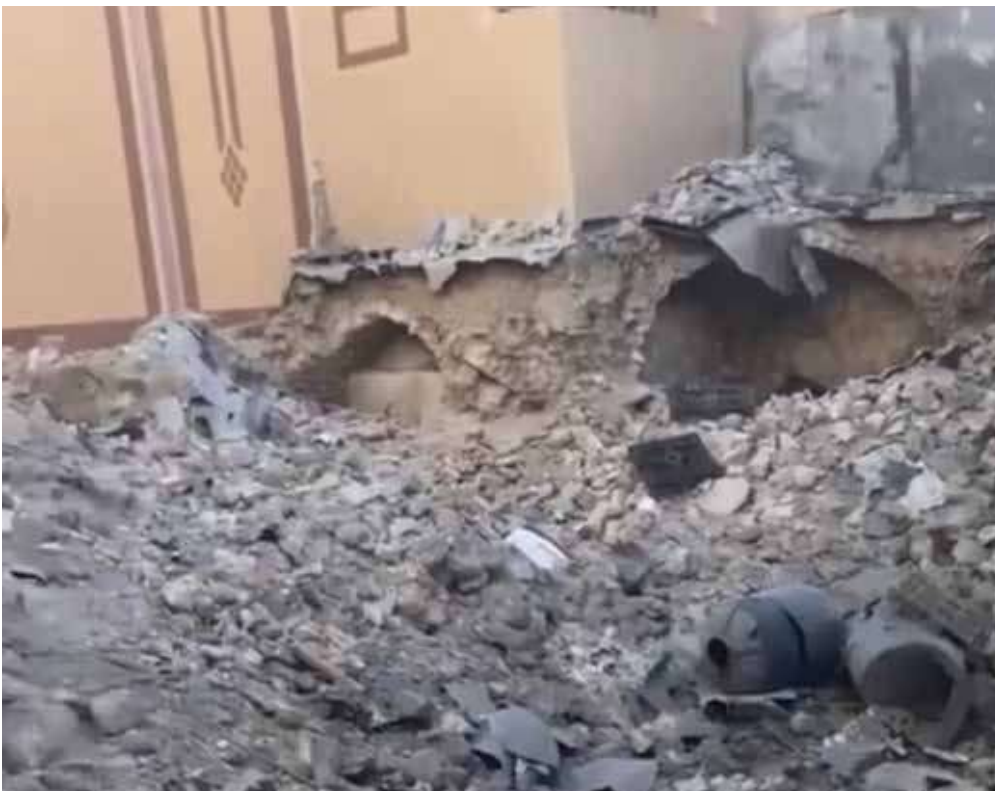
Figure 13. Hammam al-Samra, after restoration and after destruction.
